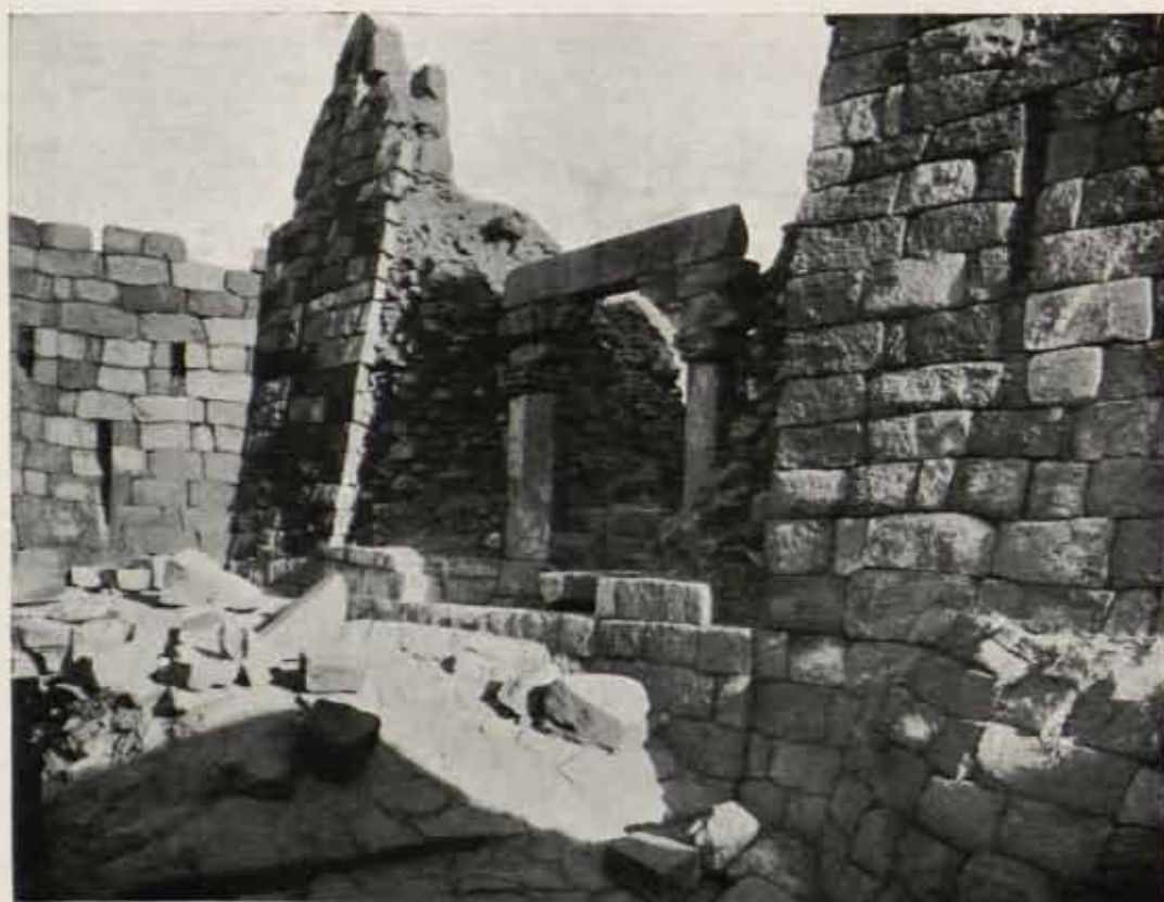
'Adilabād west gate, inner entrance before and after excavation.
